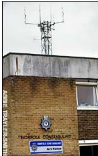
The mast at the North Walsham station
